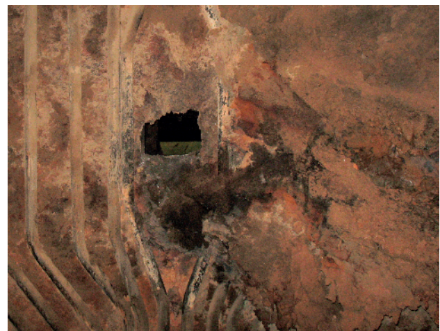
View of the same area after 12 days of operation with PentoMag® 2550 dosing.
